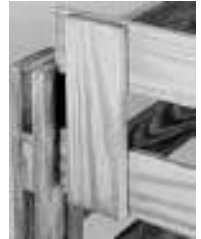
All beds are bolted together with 5" steel lag bolts for added SAFETY.
